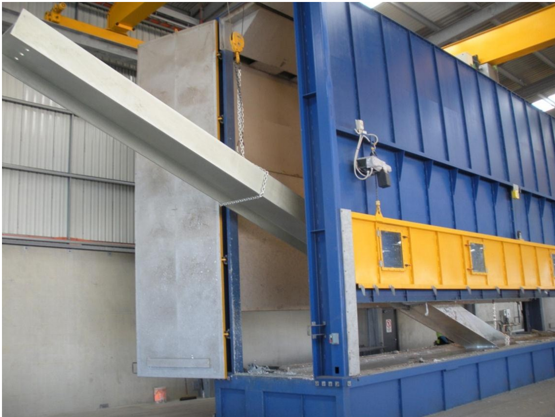
A typical zinc bath, including fume hood, showing removal of a large I beam on completion of the galvanizing process
